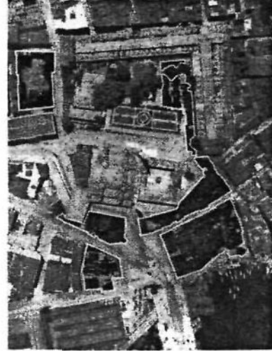
Figure 5: The areas to be demolished in Eminönü Square (Source: Güzelleşen İstanbul , İstanbul, 1943)
