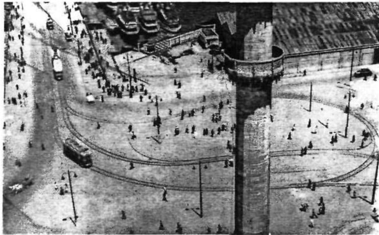
Figure 6: The Eminönü Square after the demolitions (Source: Güzelleşen İstanbul , İstanbul, 1943)
